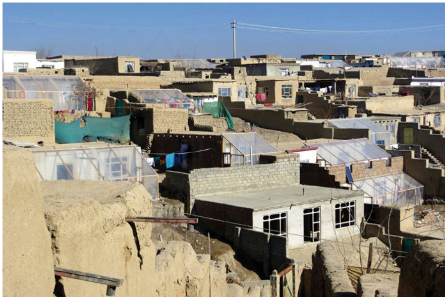
Fig. 10.1 The Passive Solar House (PSH) technology in Kabul
