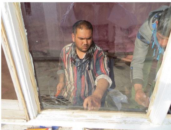
Fitting Double-Glazing
