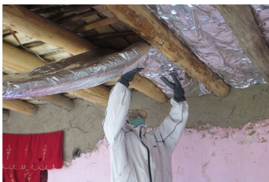
Fitting Roof Insulation
