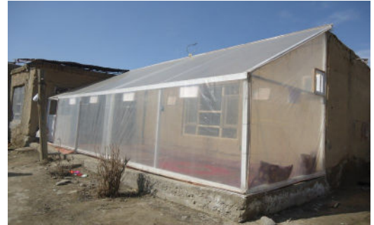
Frame covered with a plastic sheet in winter, to gain heat
