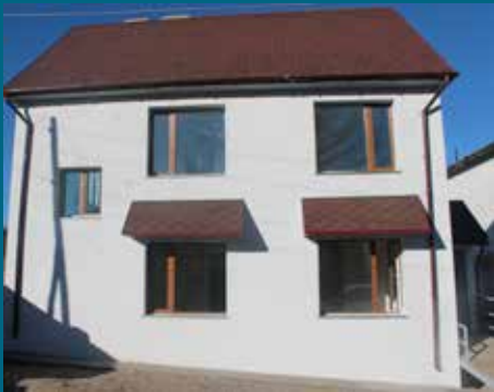
Energy efficient safe house for victims of domestic violence Tsetserleg
