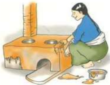
Plastering the walls of stove
