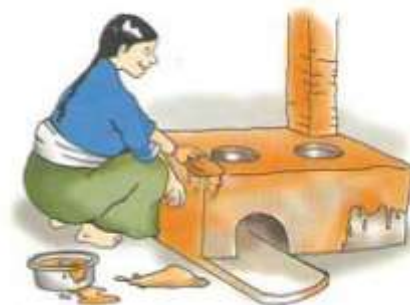
Plastering the outside surface of stove
