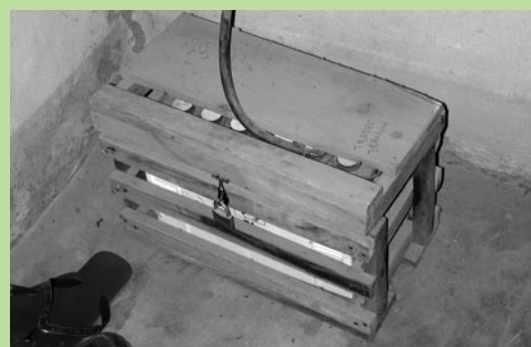
Protected battery (©SSD Yeelen Kura)
