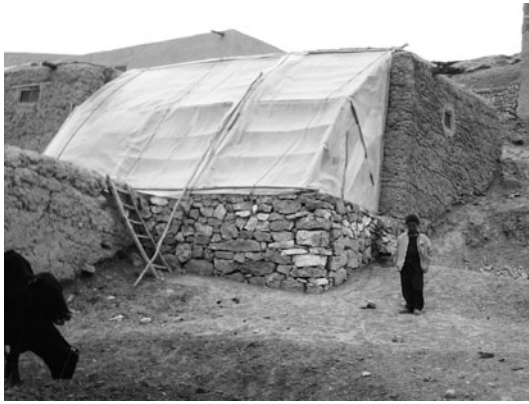
Attached greenhouse on a dwelling in Afghanistan
