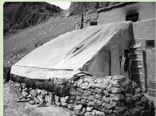
Dwelling with a passive solar system installed
