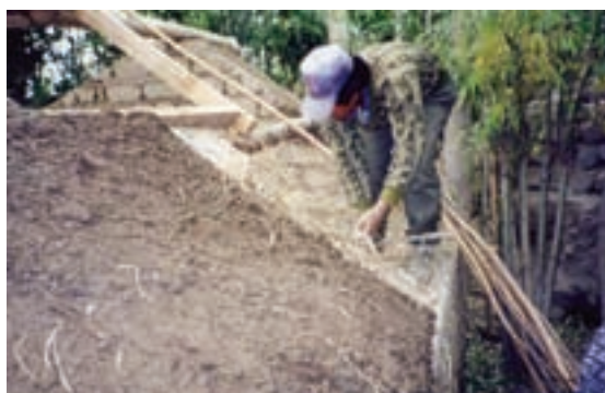
Figure 62: Applying the layers of cardboard, straw, and mud
