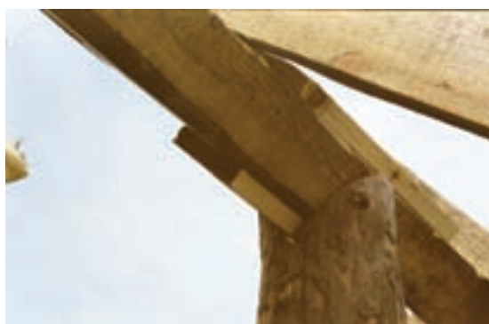
Figures 56: Fixing the beam to a post, Ladakh (top) and Qinghai (bottom)
