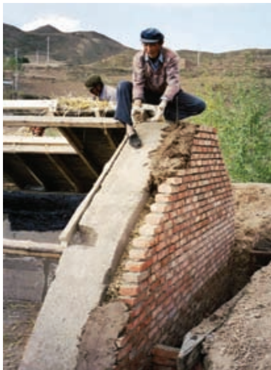
Figure 39: Construction of an outer wall with baked bricks and an inner wall with stabilised rammed earth in Qinghai
