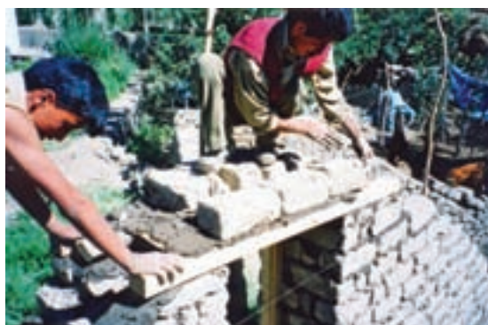
Figure 48: The masonry procedure for building the wall supporting the doorway
