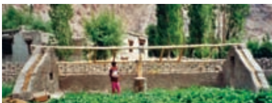
Figure 57: Roof structure with two beams and shutter frames in position in Spiti
