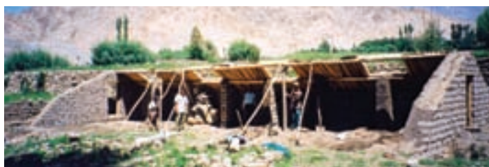
Figure 13: Greenhouse under construction (view of the double walls and the structure of the roof)
