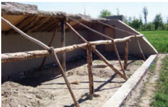
Figure 74: Wooden support structure for the polythene sheet (Lowgar, Afghanistan)
