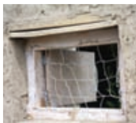
Figures 53 & 54: Inside and outside views of installed side shutter with chicken mesh outside
