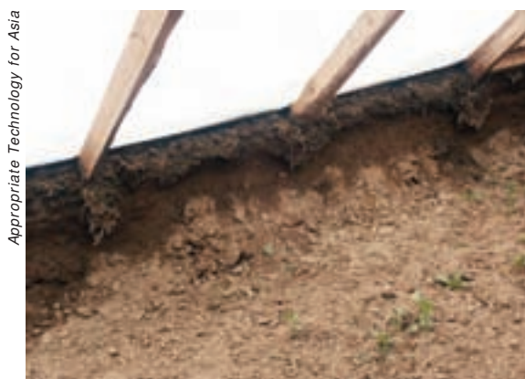
Figure 75: Joists balanced on a crumbling earth layer (outside ground level) in a greenhouse without southern foundations
