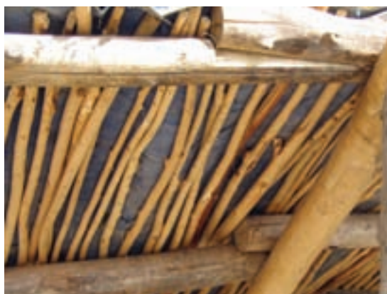
Figure 61: The layer of sticks forming the underside of the roof
