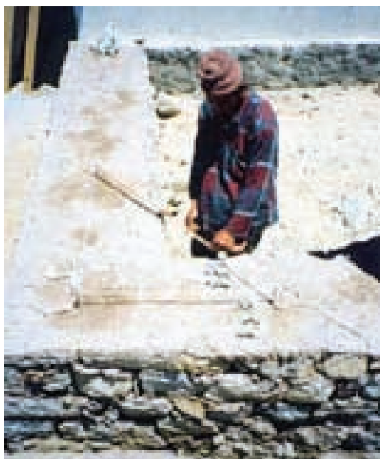
Figure 28: Drawing a right angle using the '3,4,5' method
