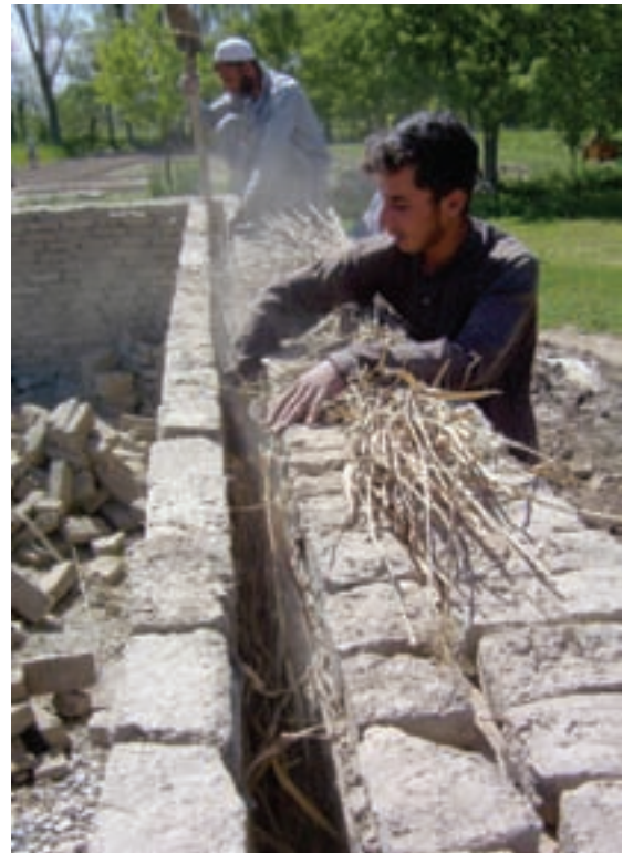
Figure 37: View of double wall separated by insulation layer (sticks are added to reinforce the gap)
