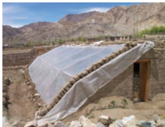
Figure 77: General view of fixing of the polythene sheet
