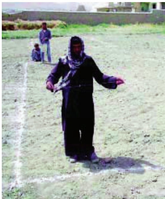
Figure 31: Marking the position of the walls
