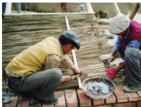
Figures 65 & 66: A roof structure made of timber and bamboo (Qinghai)
