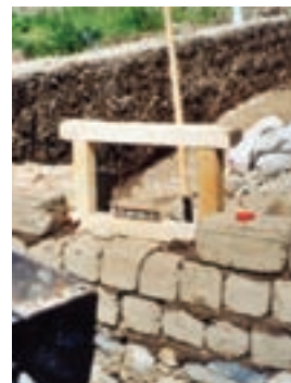
Figure 52: Positioning the shutter frame on the wall
