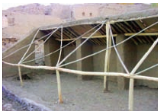
Figure 42: Completed inner partition walls, greenhouse in Zeback district, Afghanistan
