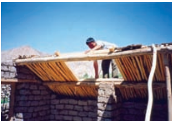
Figure 70: Fixing the frame of the roof shutter
