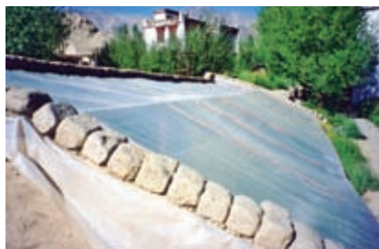
Figure 76: Close-up view of fixing the polythene sheet with mud bricks laid on a mud coating
