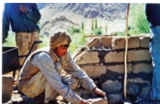
Figures 33, 34: Outlining the position of the top of the wall with thick string (in Qinghai and Ladakh)
