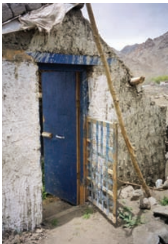
Figure 49: A second shutter covered by metal bands
