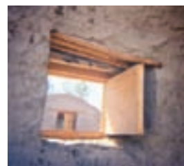
Figures 53 & 54: Inside and outside views of installed side shutter with chicken mesh outside
