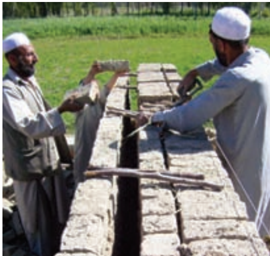
Figure 36: Building a double wall with mud bricks in Afghanistan
