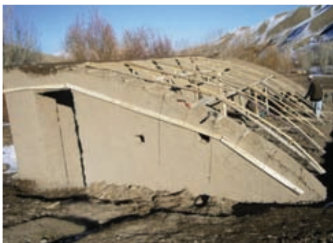
Figure 2: Constructing a greenhouse in Afghanistan
