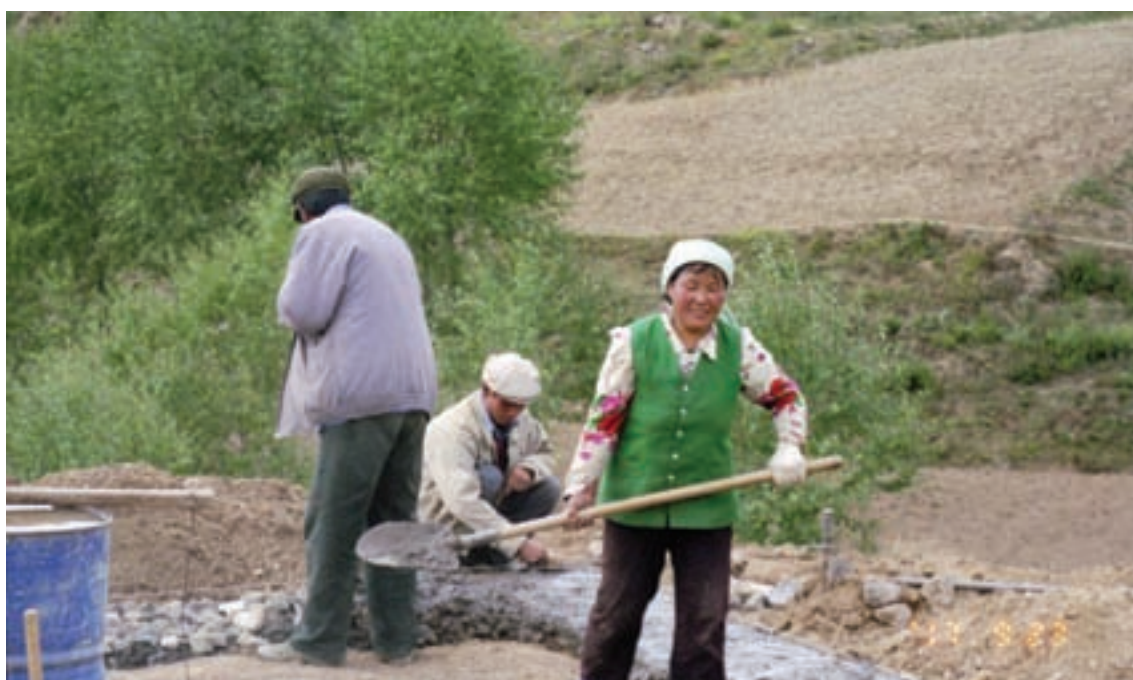
Figure 32: Covering the top of the foundation with a layer of concrete
