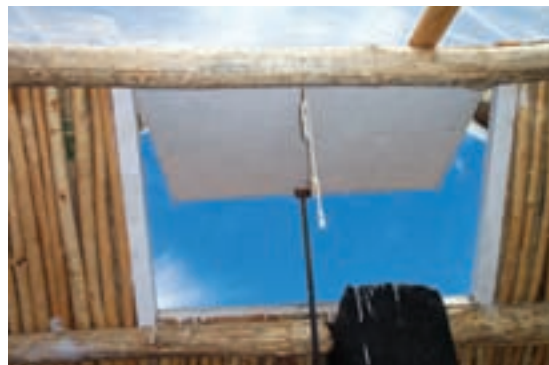
Figure 68: Inside view of the roof shutter propped open
