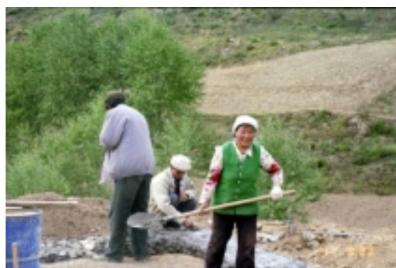
Picture 14 - A 2 inch thick layer of concrete at the top of the foundations
