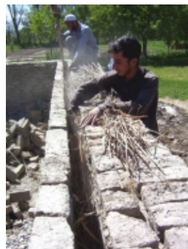
Picture 19 - View of double wall and insulation filling (sticks are added to reinforce the gap)
