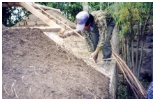
Picture 36 – Applying of cardboard, straw and Mud
