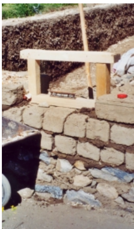
Picture 26 - Frame positioning on wall
