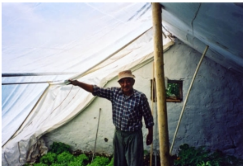
Picture 48 - View of installed night insulation
