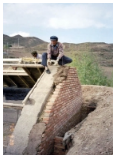
Picture 18 - Construction of the outer wall with baked bricks and the inner wall with stabilised rammed earth in Qinghai
