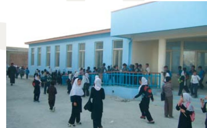
Rehabilitated school in Kabul
