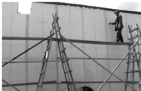
External wall insulation in Qu Deng
