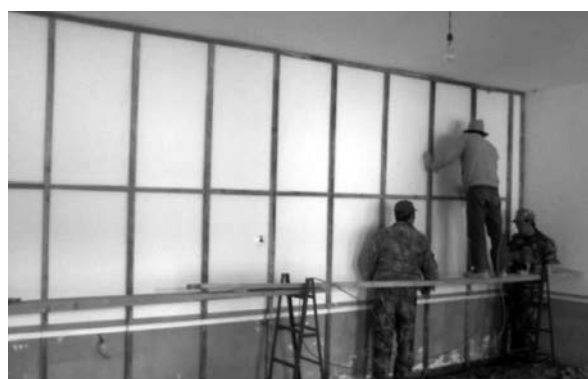
Internal wall insulation in Wu Ma
