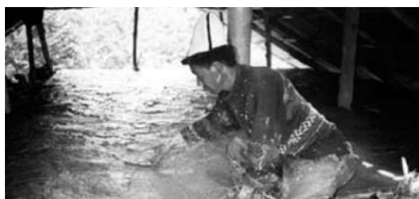
Ceilings are insulated with a layer of insulation (straw, sawdust, straw and reed, prefabricated straw and loam plates) on the garret floor which is then covered with loam.
