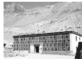
Fig 3. Solar trombe wall system Tabo monastery, Spiti
