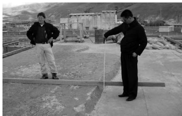
Perlite roof insulation in Yan Ba Jing
