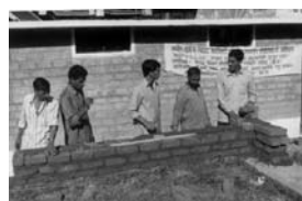
Fig 6. Training of masons in cavity wall construction
