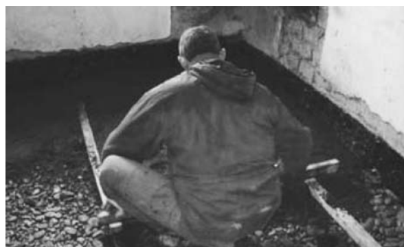
Floors can be insulated from the top, from the bottom or both. The insulation layer (straw and loam, sawdust and cotton fiber, sawdust with a hermetic covering of tar paper, prefabricated straw and loam plates, pore concrete) is put over or under the existing floor and fixed with wood.
