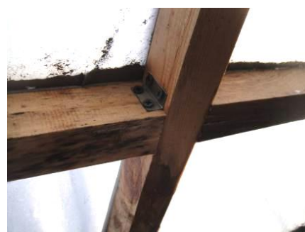
Picture 21 C: Angle brackets for south ventilation
