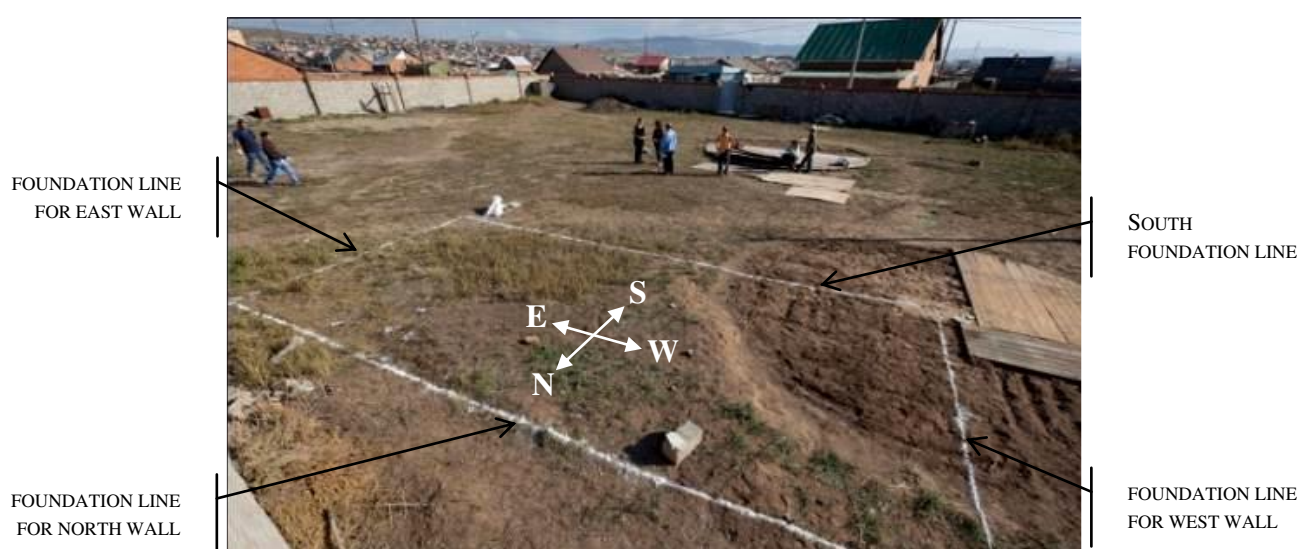
Figure 1: External foundation lines
