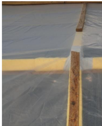
(K) Polystyrene connection between wall and roof (left). Foam below wood sticks to fix polyethylene (right)
