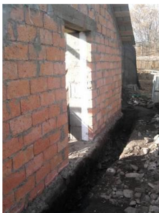
Figure 18 : Ground insulation: trench and banked earth on greenhouse side
