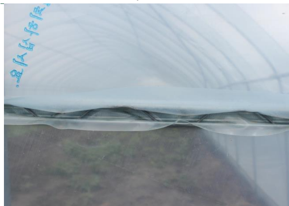
(L) Lock wire system to fix polyethylene
