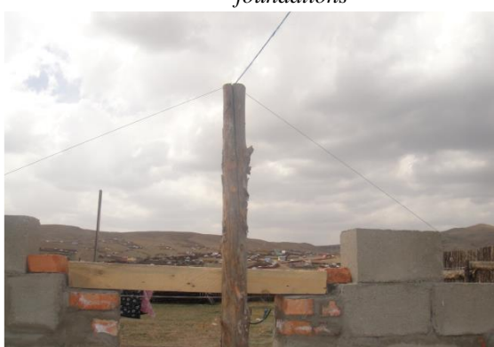
(C) Rope for wall angles and top beam
