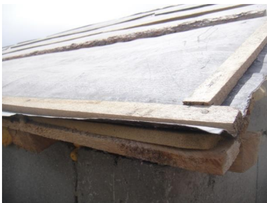
(I) Tarfelt roof and insulative thin foam layer below
