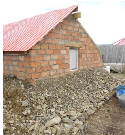
Figure 18 : Ground insulation: trench and banked earth on greenhouse side
