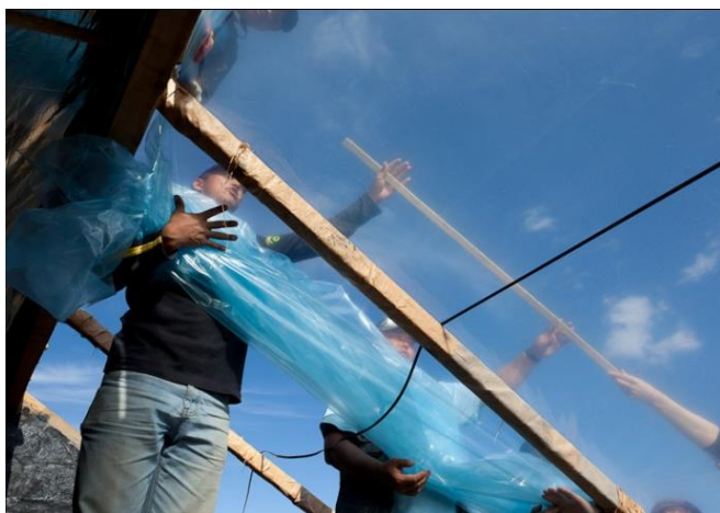
Figure 23 : Installing external polyethylene sheet
