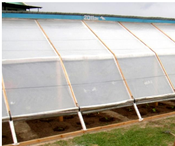
Figure 24: South ventilation and attach system
