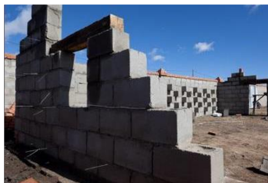
(B) Block walls, iron sticks and lintel
