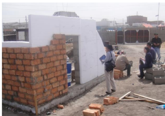
(F) Polystyrene layer and starting brick wall
