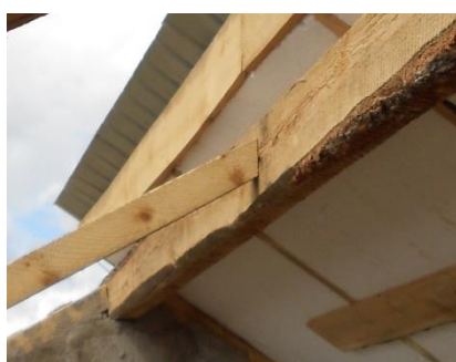
Picture 21 A: wooden joist junction on top beam
