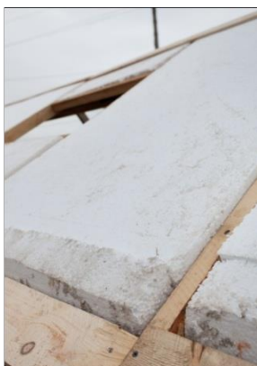
(K) Polystyrene connection between wall and roof (left). Foam below wood sticks to fix polyethylene (right)
