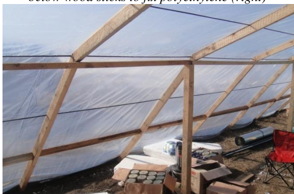
(M) Wood structure and rope to support polyethylene
