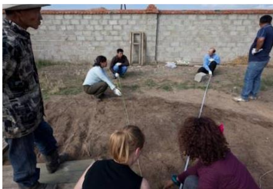
(A) Method 3-4-5 to make perpendicular lines for foundations
