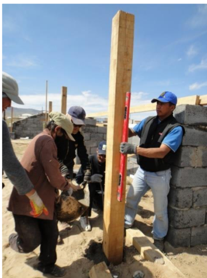
Figure 8: Central pillar: making foundations and leveling
