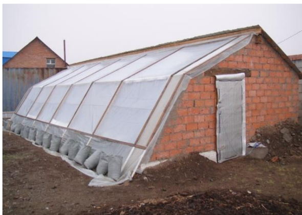
(O) Cement bag filled with sand to close south ventilation
