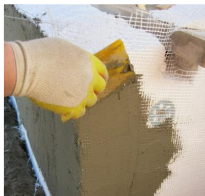
Figure 13: Protection of polystyrene with plastic mesh and plaster.
