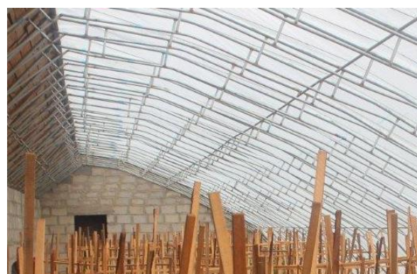
(N) Double metal structure on large chinese greenhouse
