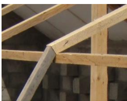
Picture 21 B: Joists junctions between lower/upper section
