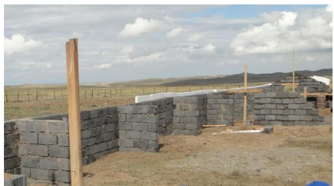
Figure 7: Inside partition walls for large greenhouse
